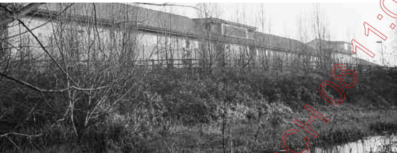
Harmondsworth Detention Centre
