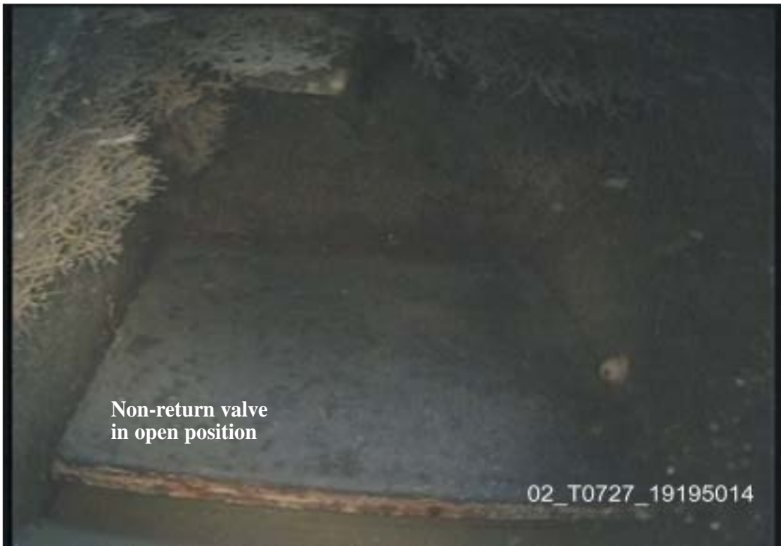
External view of opening of Offal Chute (Chute C2)
